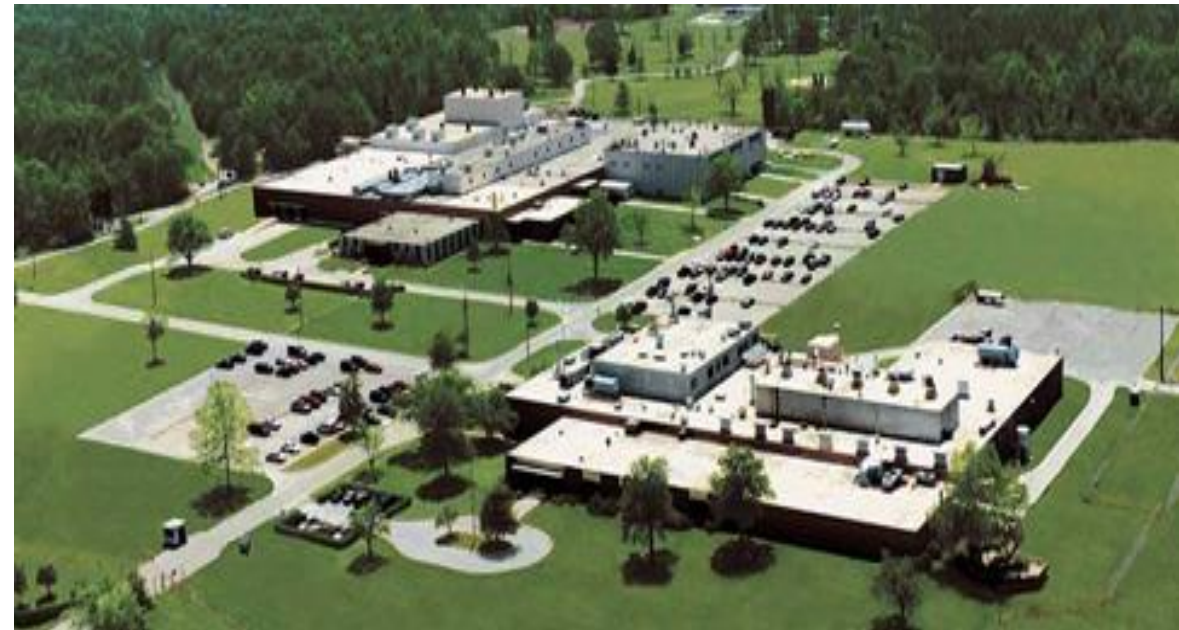
Manufacturing Plant in Laurens, South Carolina
