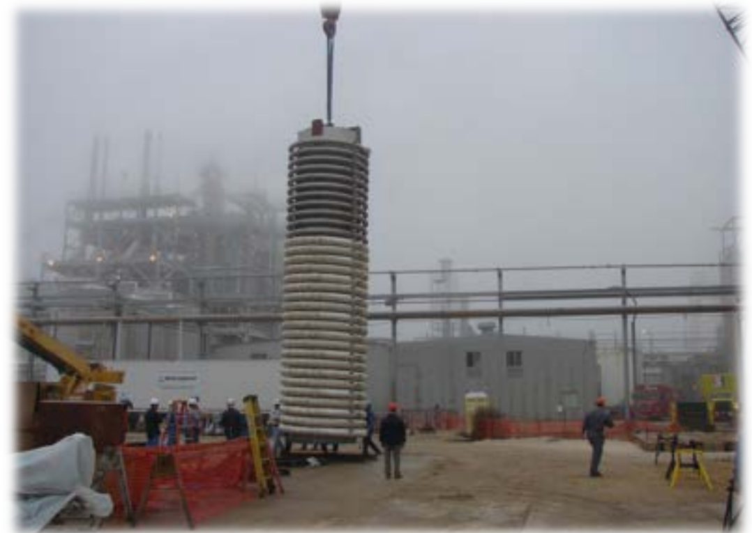
Example of installation of a 1500 kg/h catalyst treatment line
