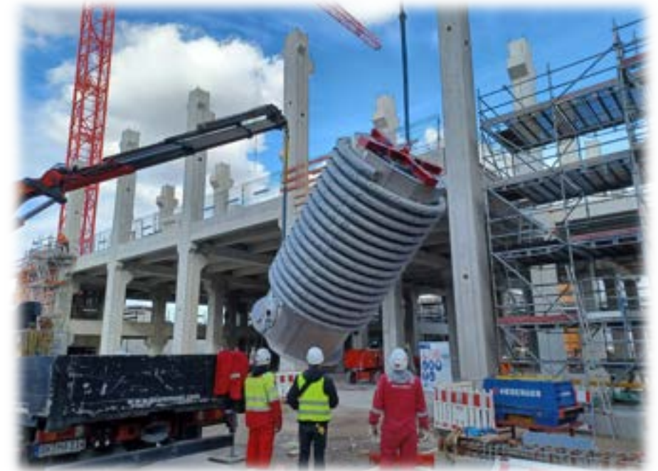
Installation of a 500 kg/h drying unit
