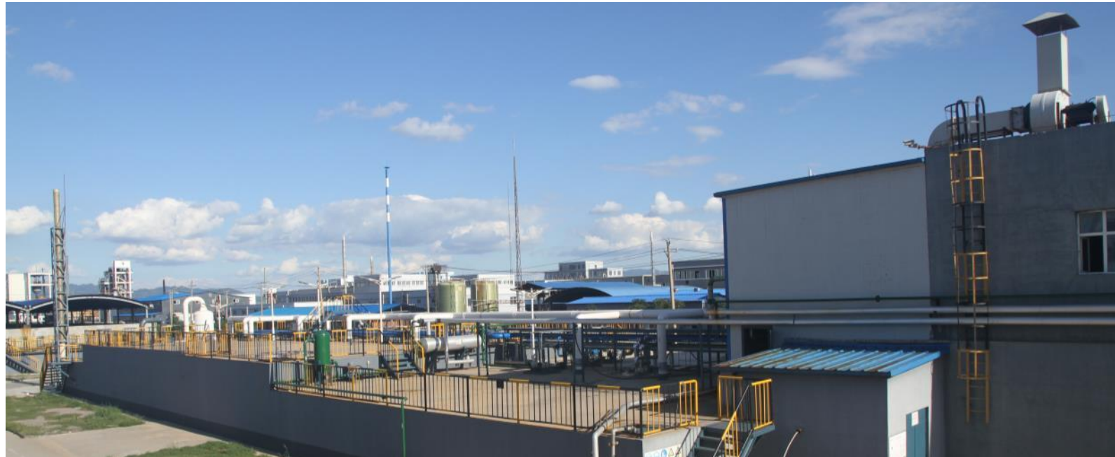
Waste Water Plant
