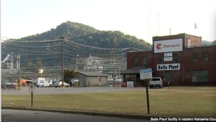
Belle Plant facility in eastern Kanawha County.
