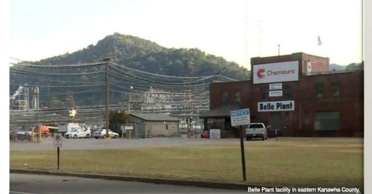
Belle Plant facility in eastern Kanawha County.
